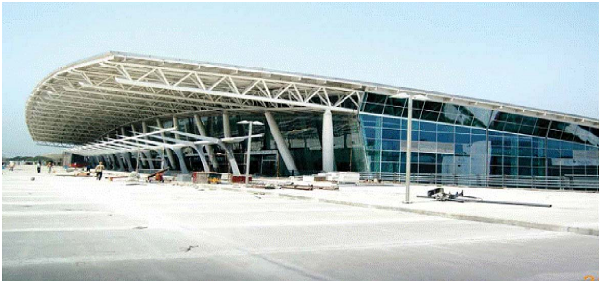
Long span trusses
