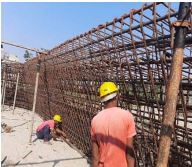
Intake Structure at Bhagalpur
