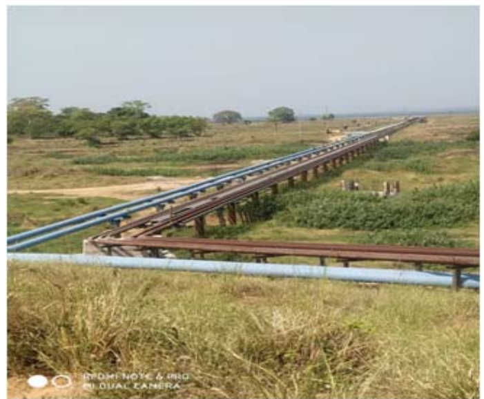
AWRS Plant at Odisha
