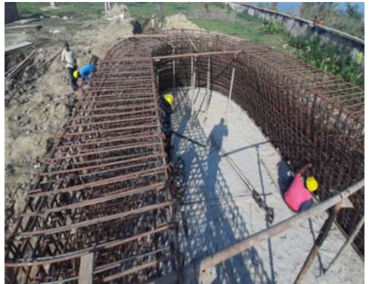
Intake at Bharalpur
