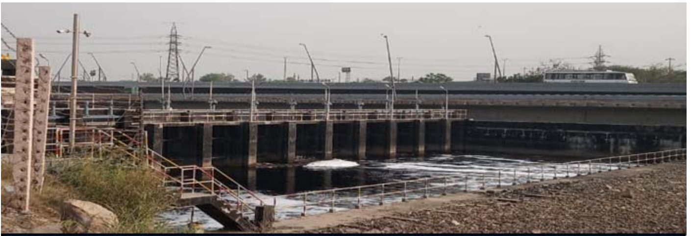
SPL-11 Interceptor Sewer Along Najafgarh, Package-3
