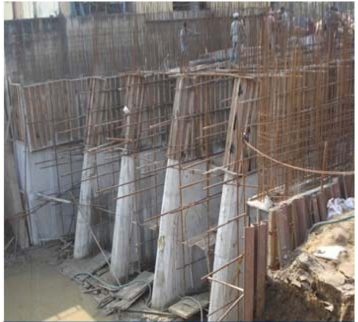
INTAKE STRUCTURE ON RIVER SIDE OF DAMODAR
