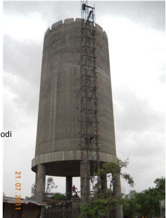
1500 ton RCC and 300 ton M.S. Ash Silos at
