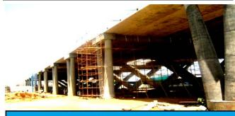
RCC precast girders with cast in situ deck slab superstructures
